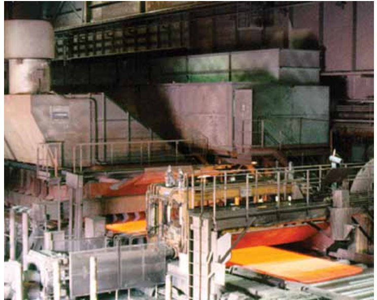
Burns Harbor 160" Mill Accelerated Cooling Unit
